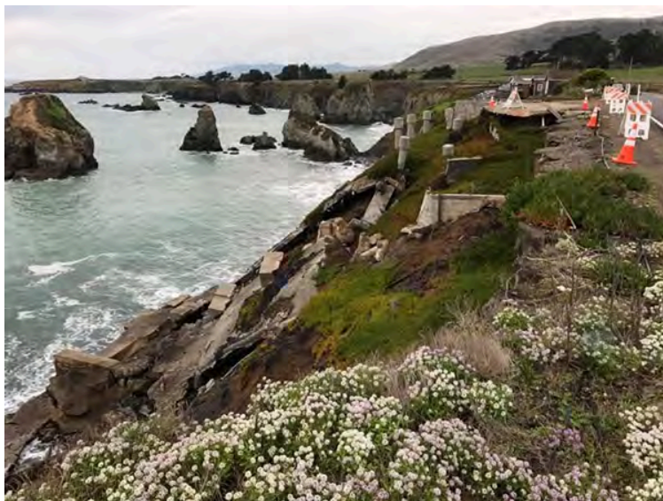
Erosion affecting SR 1 in Sonoma County, CA, where Caltrans is pursuing realignment. Source: Caltrans.
