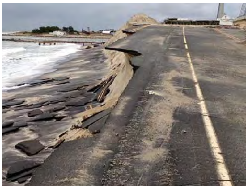
Road damage from Hurricane Sandy in Delaware. Source: Delaware Department of Natural Resources and Environmental Control.
